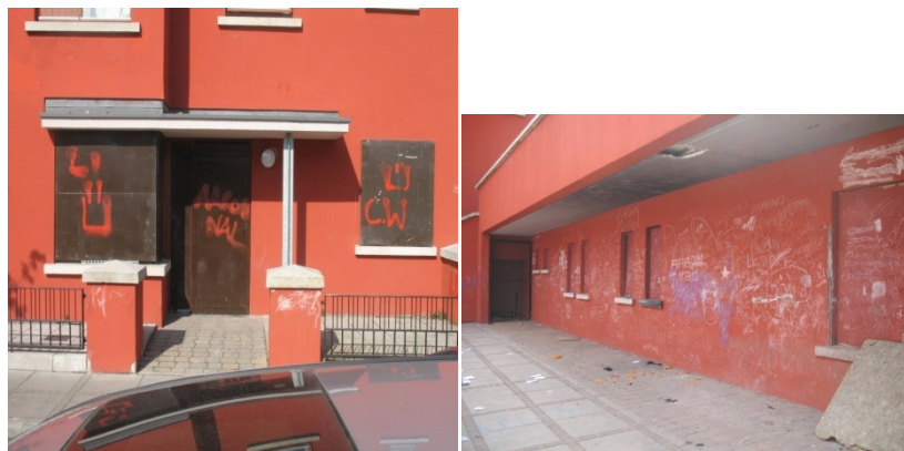
Community Centre Meile An Ri not in operation.
